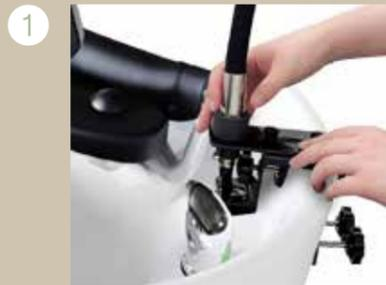
1 Completely insert the device in an easy-to-use direction, ensuring there are no gaps, and tighten the fixing screws to secure it to the ceramic.
